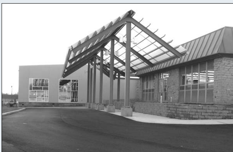
The completed circle driveway entrance. The awning is in place to protect clients in times of inclement weather.
