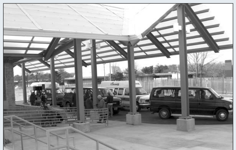
The circle driveway entrance is pictured during the busy 4 p.m. pick-up. Vans are assigned an arrival time to help organize traffic flow.
